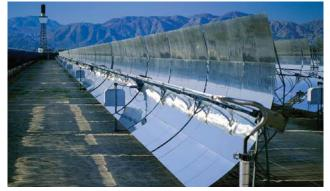
Solar-thermal parabolic trough power plant
